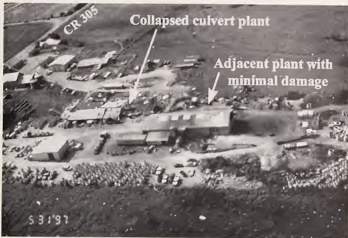
Figure 8. Aerial view of entire culvert plant complex.
