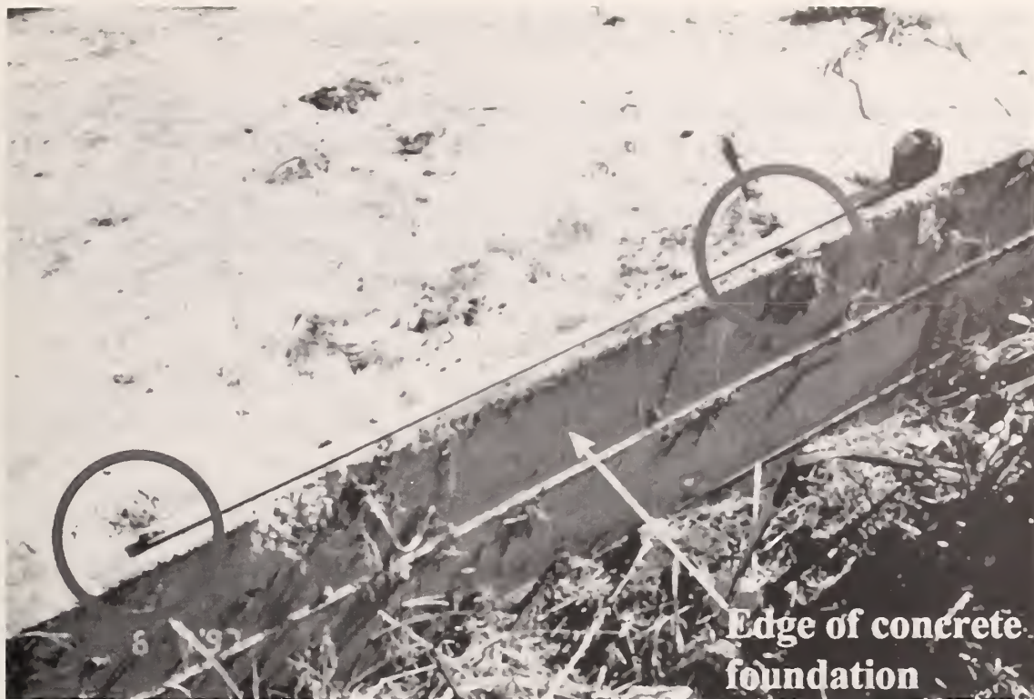
Figure 13. Evidence of pullout of nails used to fasten sill plates to concrete foundation.
